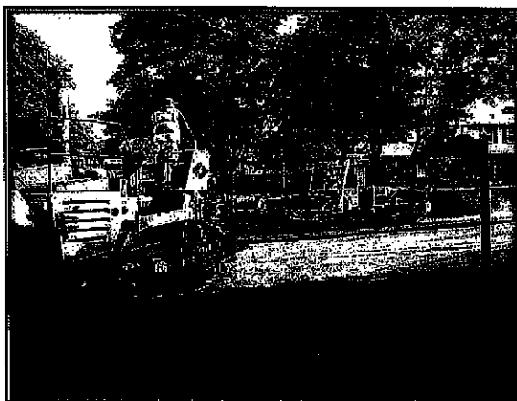
Crew leveling sub base of the road before placing asphalt.
